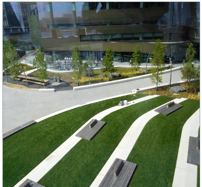
A popular feature in today's hardscapes involves precast concrete custom seating in the form of seat walls and stepped configurations, such as what was installed at Cornell Tech, located on Roosevelt Island in Manhattan, New York City. Design and photo courtesy of James Corner Field Operations
