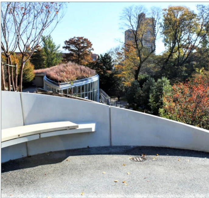
Originally, the Robert W. Wilson Overlook in Brooklyn Botanic Garden called for cast-in-place seating walls. Planners looking for a value-engineered alternative determined precast concrete provided the garden with curved seating that had a better architectural finish and was cheaper to produce. Photo courtesy of Southside Precast Products
