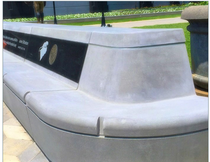
Another method to discourage skateboarders from riding on built-in seats is to incorporate recesses in the concrete rather than adding something that protrudes. Photo courtesy of Lucas Concrete Products
