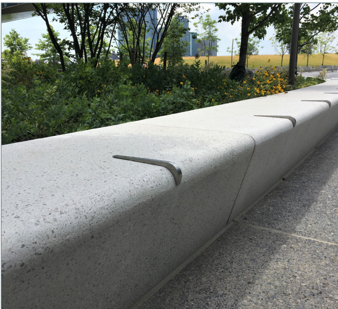
One of Sun Precast’s recent projects involved polished concrete benches — to the tune of 45 truckloads — for Cornell Tech in Manhattan. The ones here are equipped with metal skateboard deterrents. Design and photo courtesy of James Corner Field Operations
