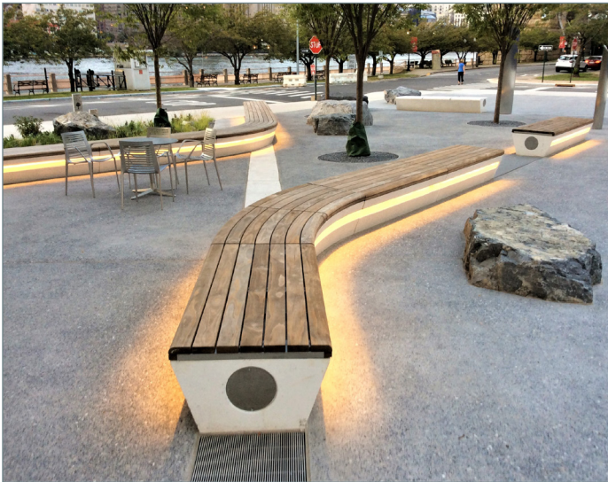
Lighting integrated into benches made with precast concrete and wood by Sun Precast help to illuminate areas at night at Cornell Tech. Design and photo courtesy of James Corner Field Operations
